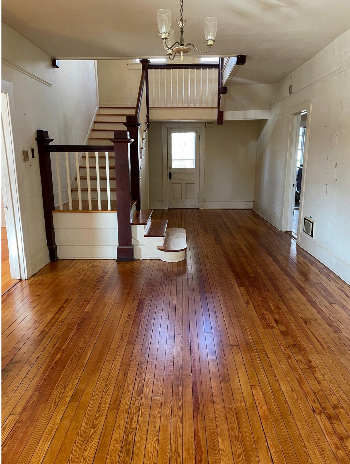
Figure 35 Central Breezeway Foyer. Narrow 2 1/2" Heart Pine Flooring Considered to be Esthetically Superior to the 3 1/4" Yellow Pine Flooring Found in the Rest of the House. A public greeting area. The Grandest Room in the House.
