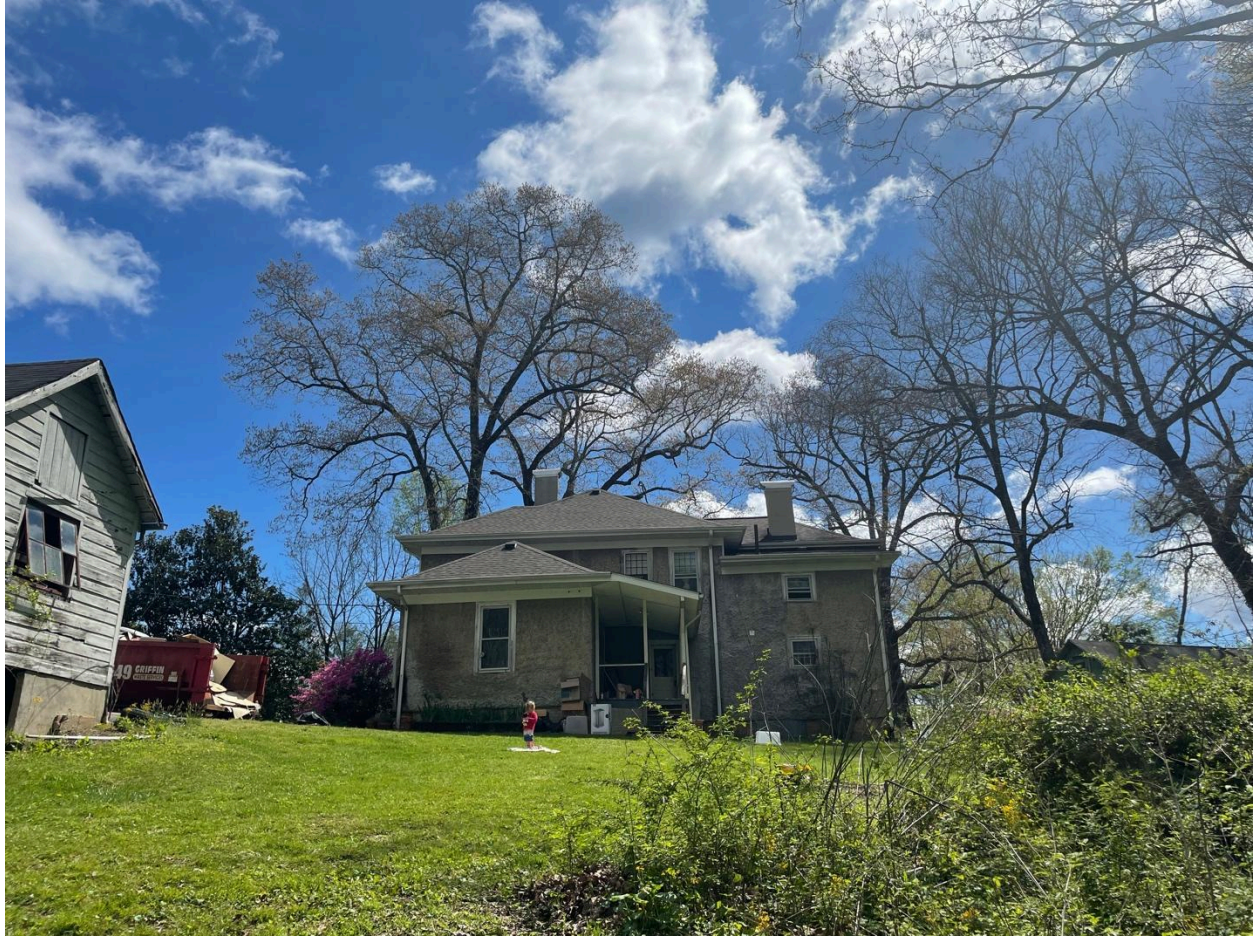
Figure 20 West Elevation Rear of House. Clapboard Sided Outbuilding Exhibits Six-pane Steel Casement Windows and Hinged Opening Above.
