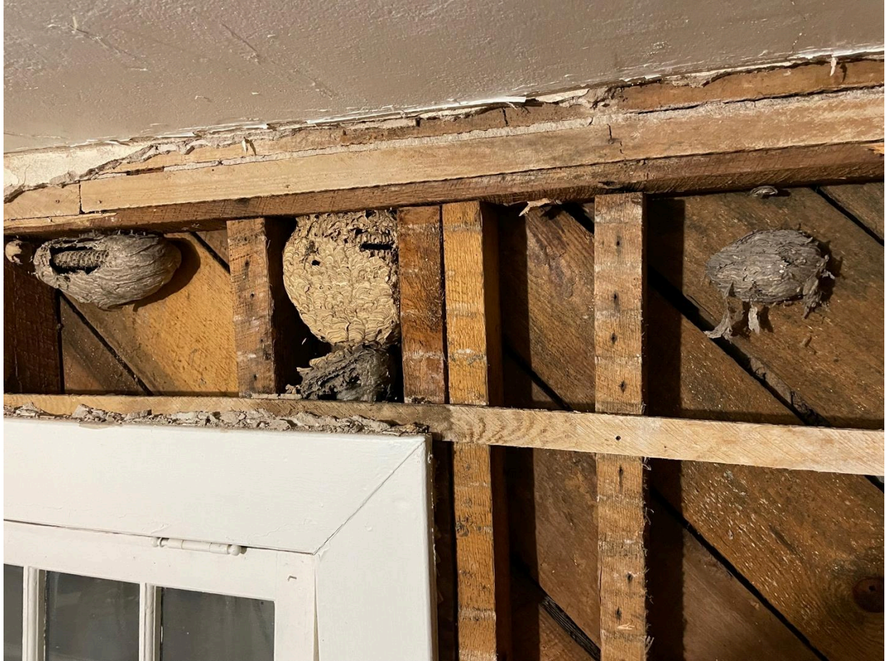
Figure 22 Wide Hand Hewn Exterior Sheathing Planks Various Dimensions, Proper 2" x 4" Hand Hewn Lumber Studs, and Resident Aviators.
