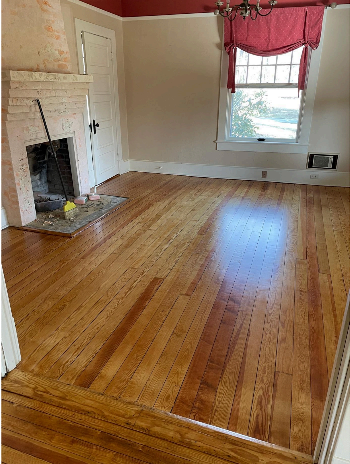
Figure 34 Double Pocket Door Reveals Sitting Room with Original Brick Fireplace. Fireplace Contains Single Chimney with Double Flue for Dining Room Fireplace.
