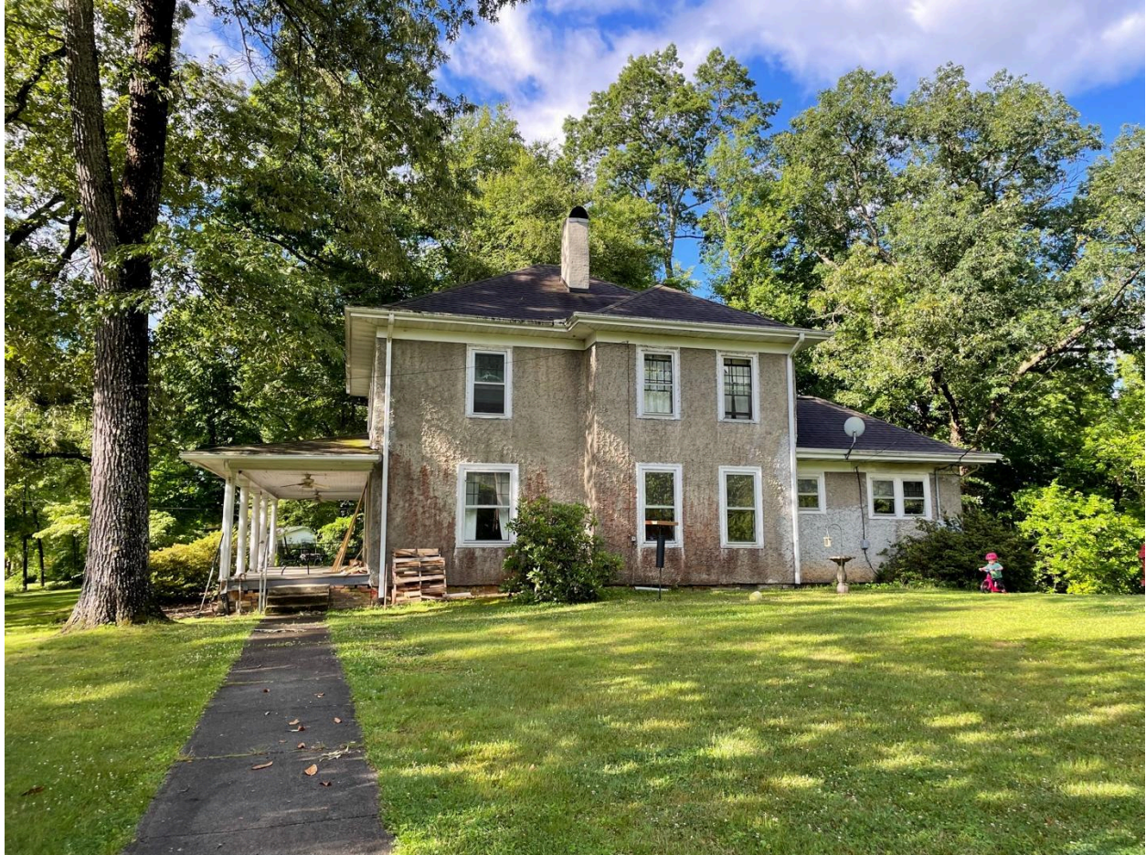
Figure 18 North Elevation. Mature White Oak Far Right Over 150 Years Old. Mature at Time House was Built. Described in 1916 Deed as 48" White Oak. Massive. Per NC Forester Jordan Luff, Habit Suggests it was "Open Grown."
