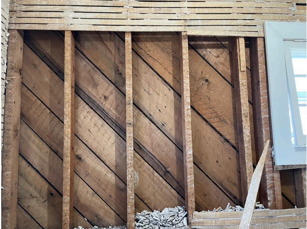
Figure 23 Lath and Plaster Walls with Hand Hewn Irregular Width Planks with Pebbledash Siding Beyond Allows the House to "Respire" Over the Seasons. For Better or Worse.
