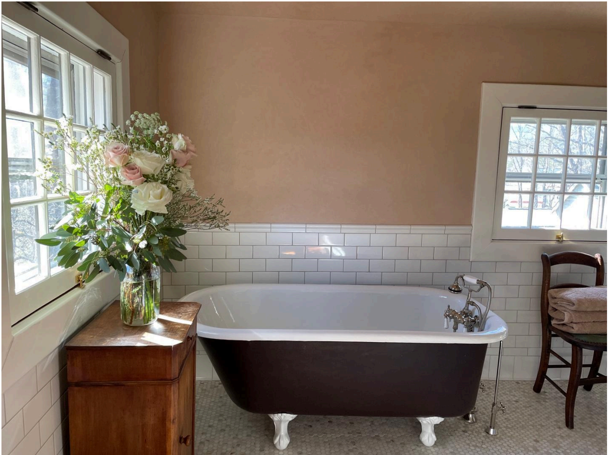
Figure 39 Original Claw-and-Ball Foot Tub Restored with Fresh Enamel and Paint.
