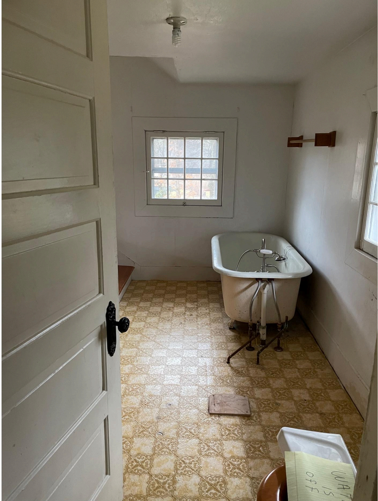
Figure 37 Original Clawfoot Tub with Telephone and Swanneck Faucet. Original Mortis and Tennon Twelve Pane Casement Windows.
