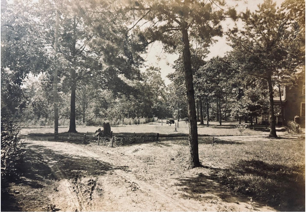
Figure 6 Southbound Present Day Carolina Avenue.
