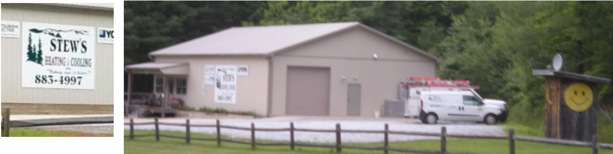
Stews Heating & Cooling: 6837 Greenville Highway
