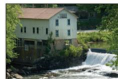
**25 Dillsboro Dam and Power House.** Possibly the smallest powerhouse in the US, the dam has generated electricity since 1913. The station includes a concrete dam 12' high and 230' long, with a metal sheeted powerhouse.
