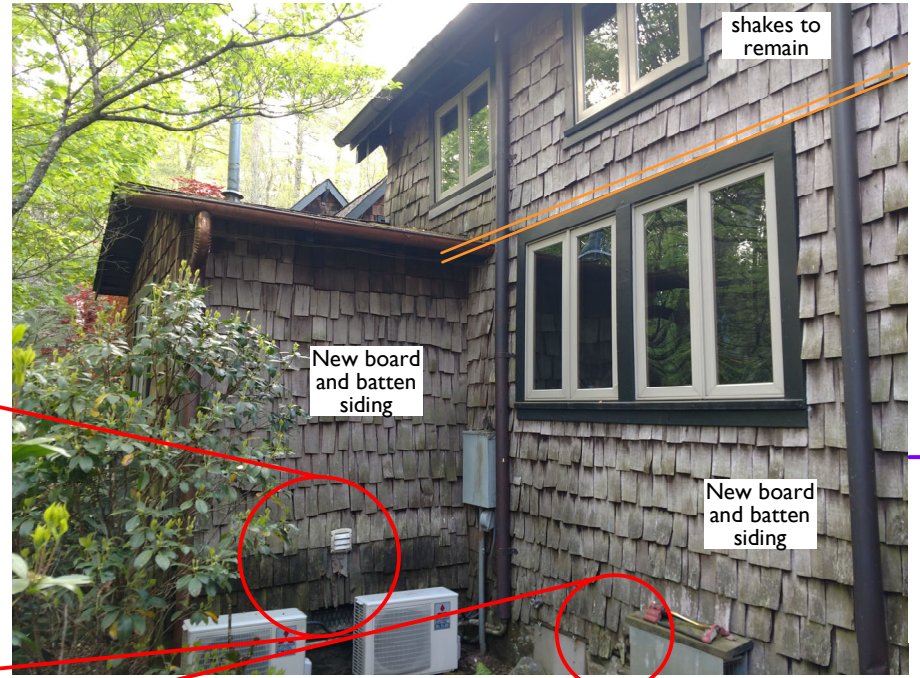
Deteriorating Chestnut Shakes in need of replacement
